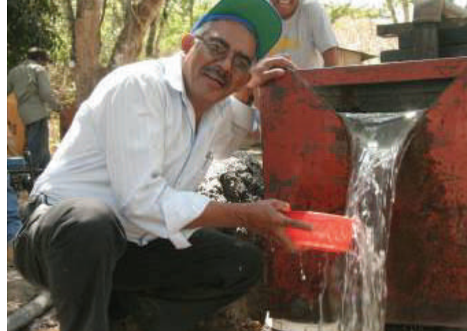
Pastor Miguel Duran at the drilling site
